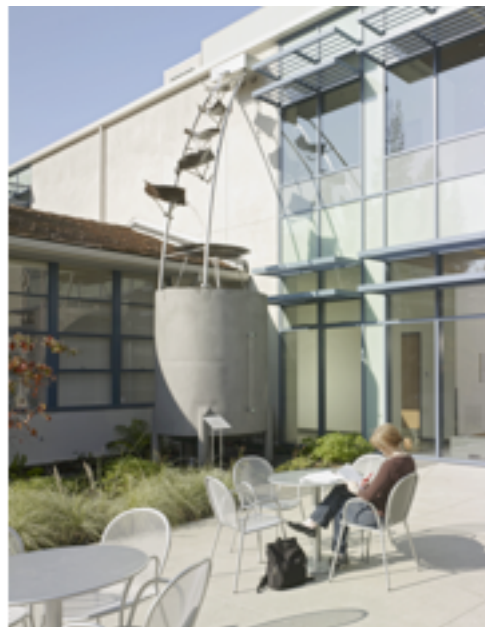
Mills College Natural Science Building Rain Catchment Fountain
